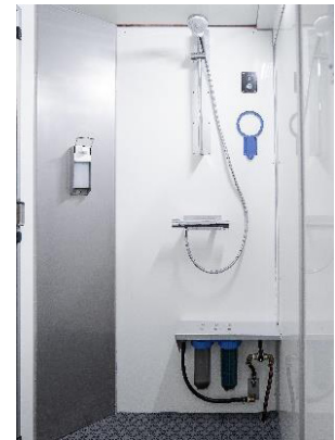
Shower with 2-stage wastewater filtration
