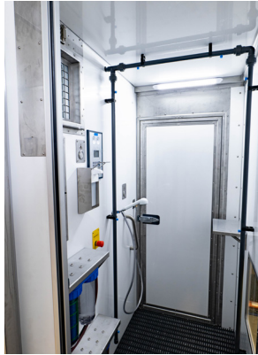
Negative pressure disinfection area with shower and spray disinfection
