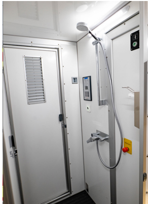
Shower with 2-stage wastewater filtration
