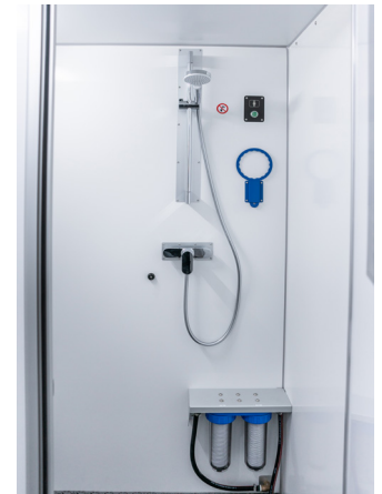
Shower with 2-stage wastewater filtration
