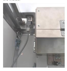
Connect the supplied electrical cables to the three connections on the outside of the roof (where the plugs are also connected from the inside) and connect them to the forced locking control unit. It does not matter in which order the three plugs are connected to the control unit.
